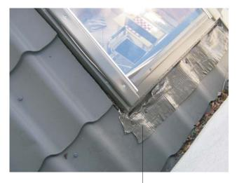
Badly fitted/ damaged — Velux flexible flashing
