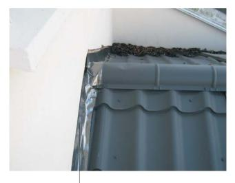
Adhesive tape flashing peeling off wall
