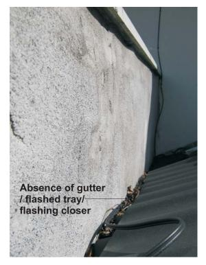
Photo looking in at parapet wall
