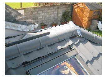
Adhesive tape flashing \_\_\_\_\_\_ peeling from capping junction
