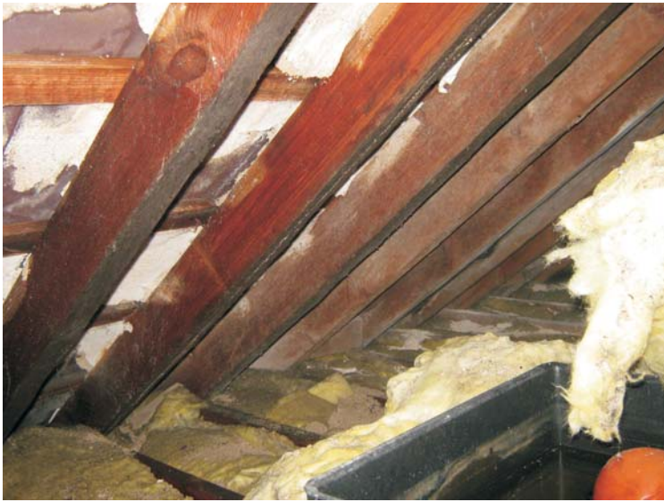
Photo 7 - saturated rafters
