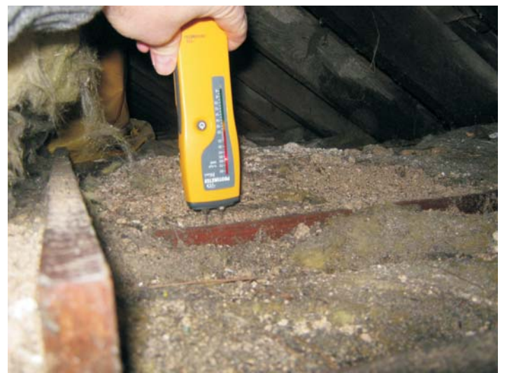
Photo 4 - joist 80% moisture
